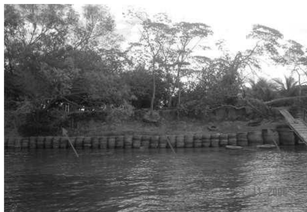
Figure 8. Protection of the island with tires. The arrows highlight the trees falling along with portions of the ground that support them.
